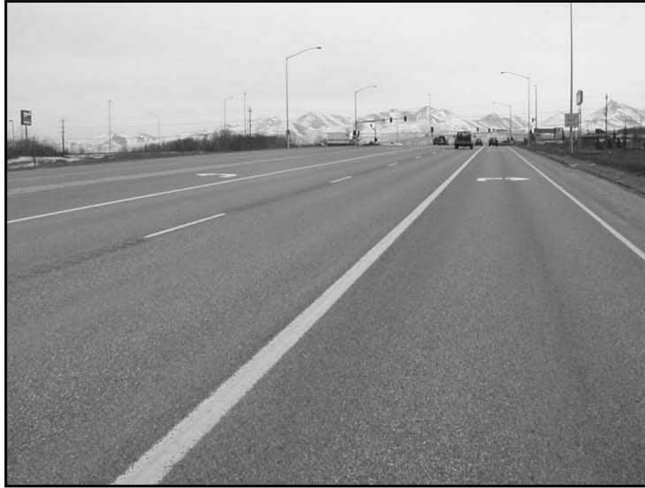
Photo 2.17: Anchorage SMA, PG-64-28, heavy truck traffic area, 4 years old, ~ 0.4-in rut
