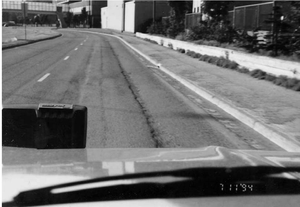
Photo 2.10: File photo of Egan Drive in Juneau, Type II mix prior to Superpave
