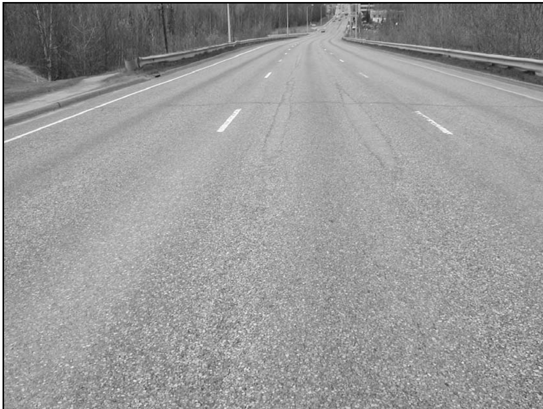
Photo 2.23: Worn through areas in 1985 Anchorage Plus Ride mix
