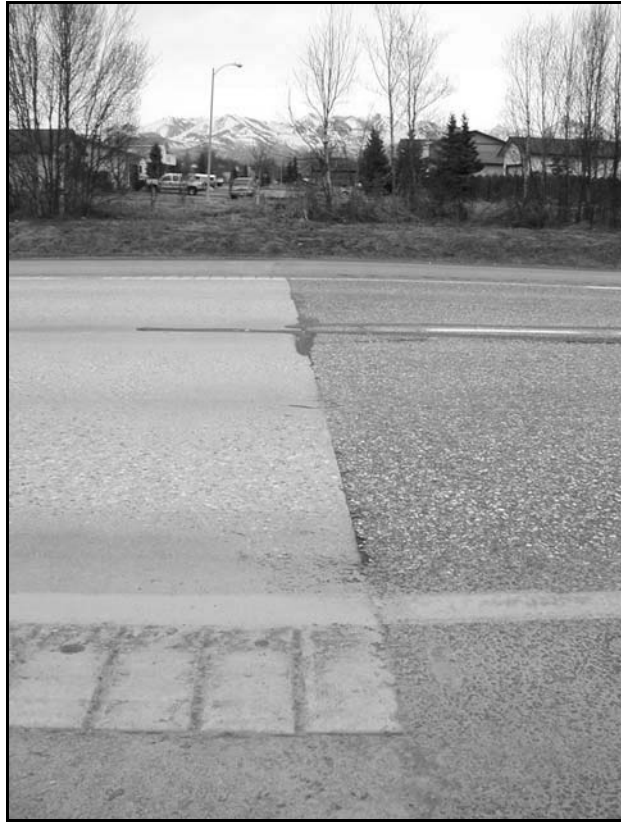
Photo 2.19: Upstream edge of Anchorage WIM slabs with adjoining SMA with PG58-28
