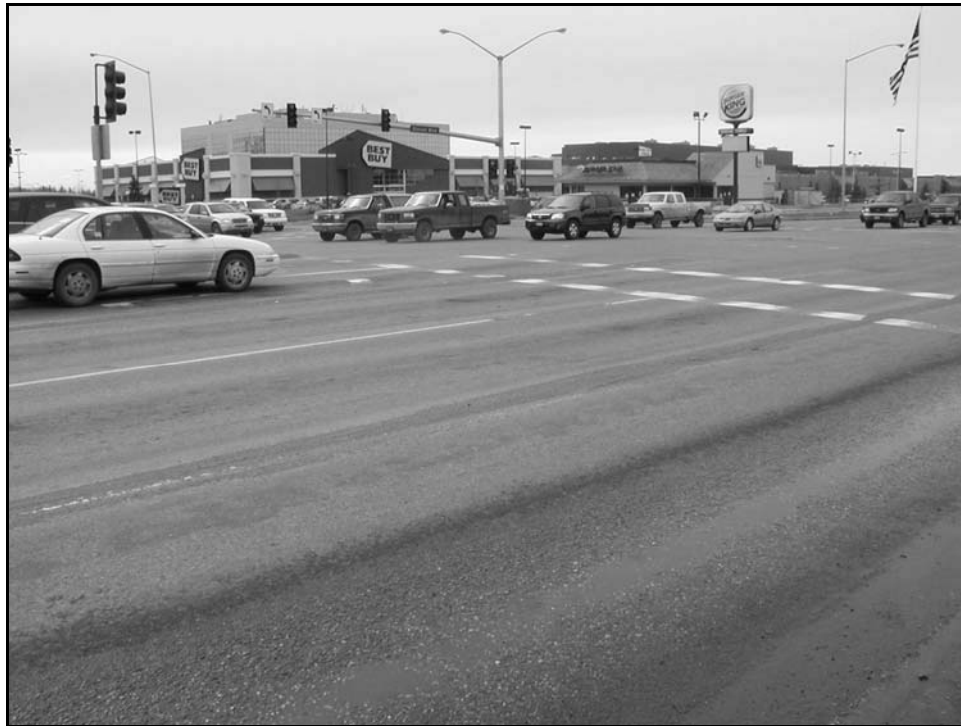
Photo 2.15: SMA with PG58-28, 2-year old mix in Anchorage with +0.3-in ruts
