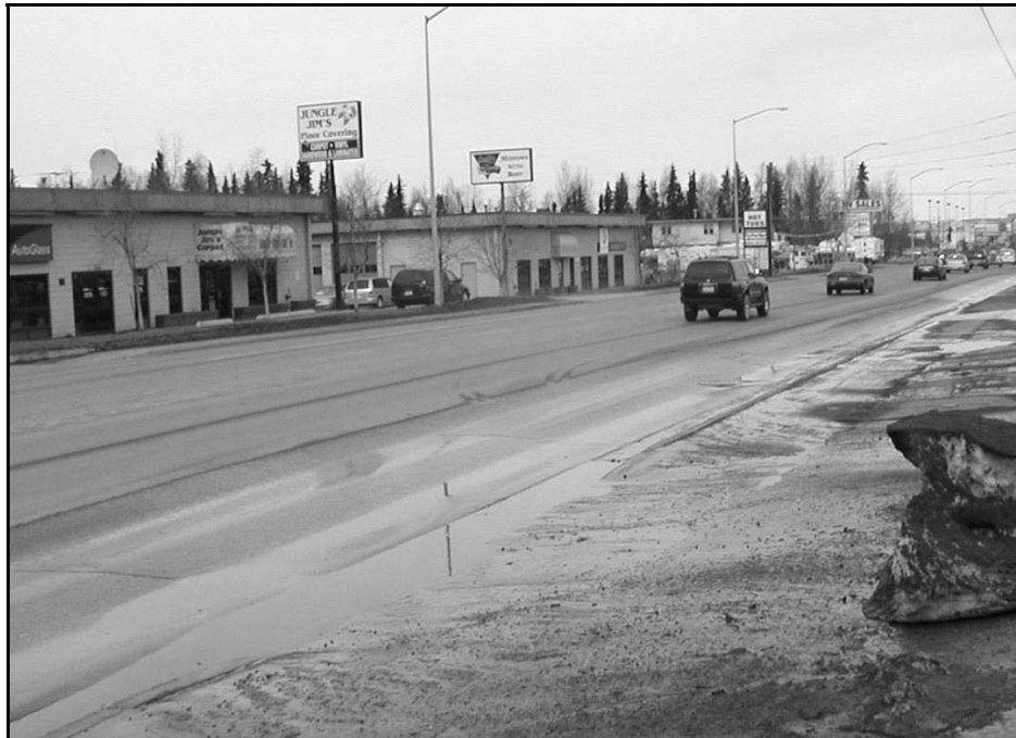
Photo 2.5: Asphalt Concrete, Type II placed in 1994
