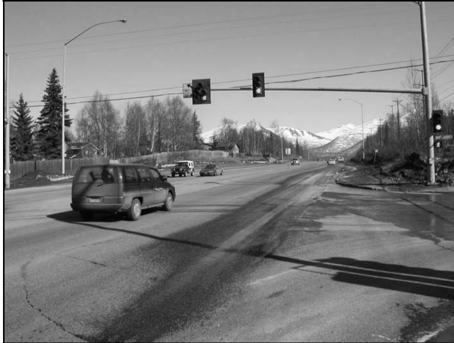
Photo 2.14: 7.5 year old SMA with AC-5 with +0.5-in ruts - Anchorage
