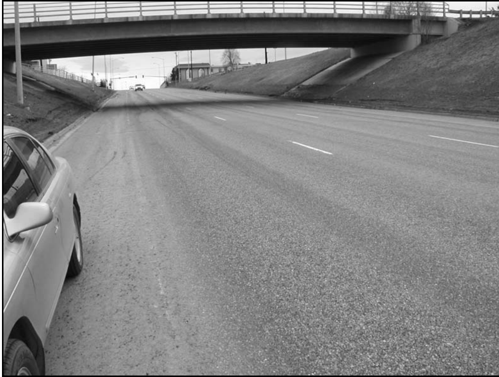
Photo 2.22: Anchorage Plus Ride mix placed in 1985 still performing well
