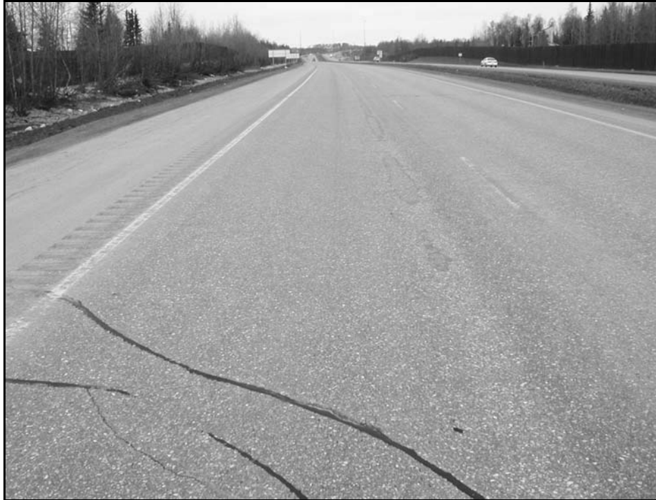
Photo 2.4: Anchorage Asphalt Concrete, Type II overlay placed in 1982
