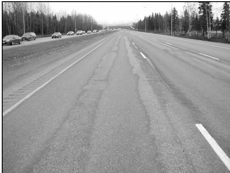
Photo 2.7: Anchorage studded tire wear on Type III overlay mix (< 1 year old)
