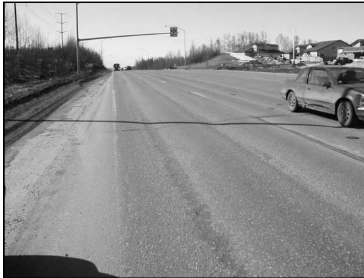
Photo 2.1: Anchorage Type I mix overlay, nearly 13 years old.
