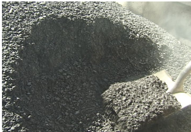
Asphalt mixture in a haul unit
