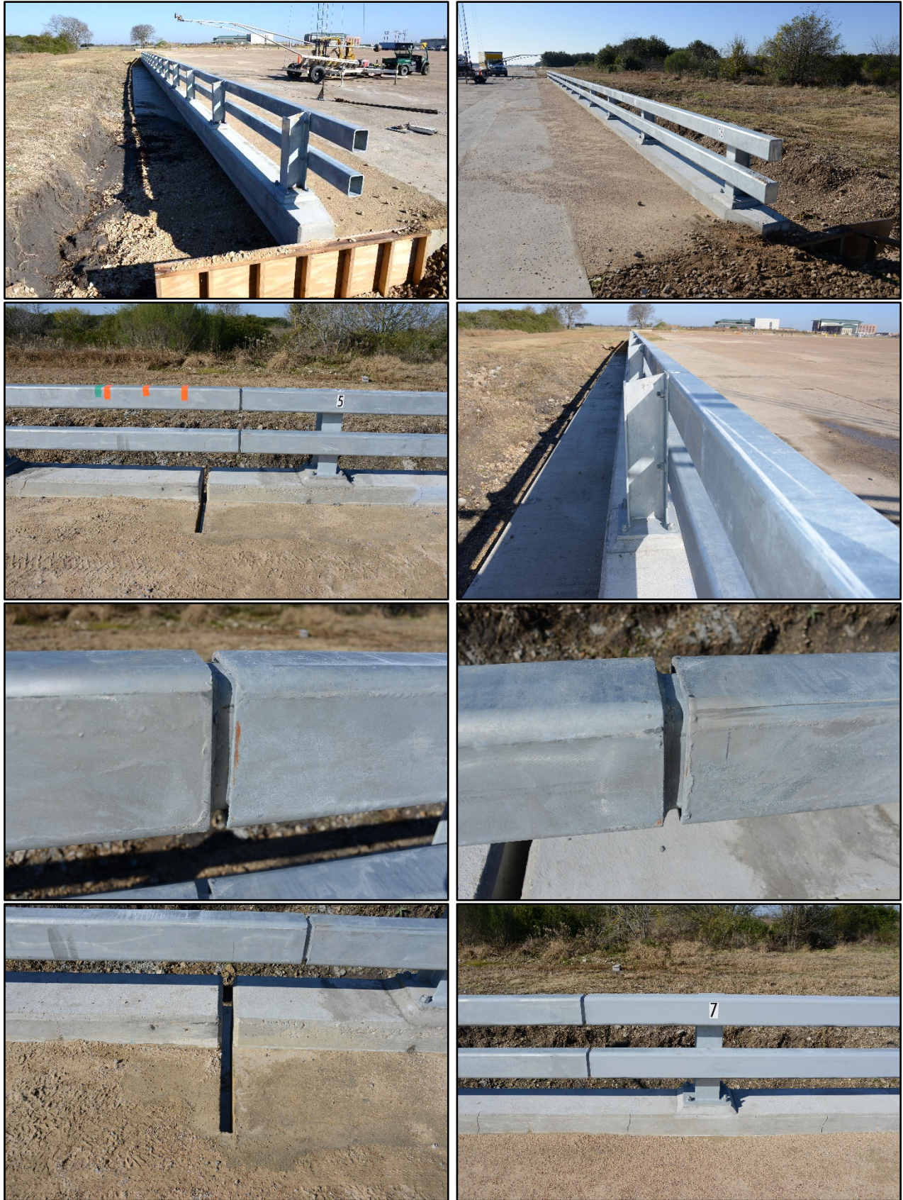
Figure 2.2. 2019 MASH 2-Tube Bridge Rail prior to Testing.
