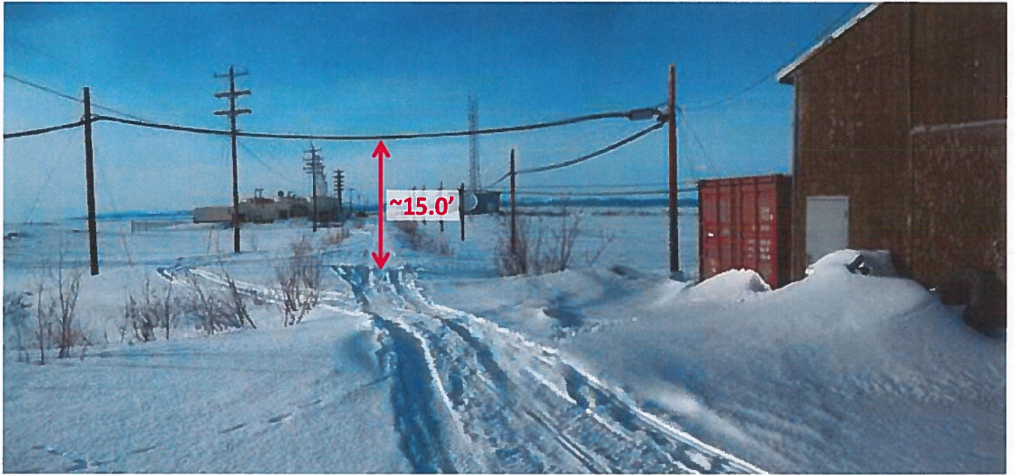
Near "BL" 10+40 looking north on Barge Landing Access Road. Clearance is existing.
