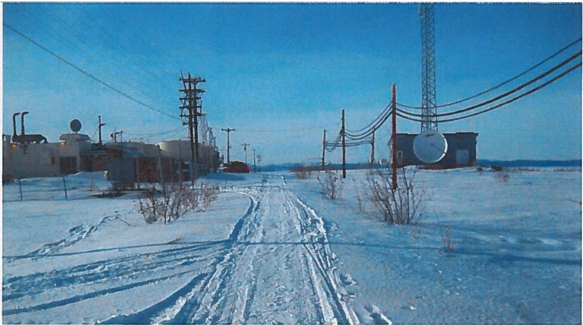
Near "BL" 14+40 looking north on Barge Landing Access Road
