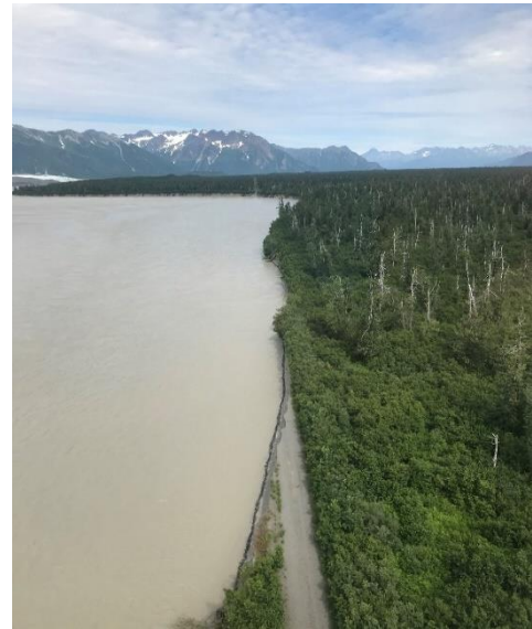
Photo 1. Washout, CRH MP 44-45
