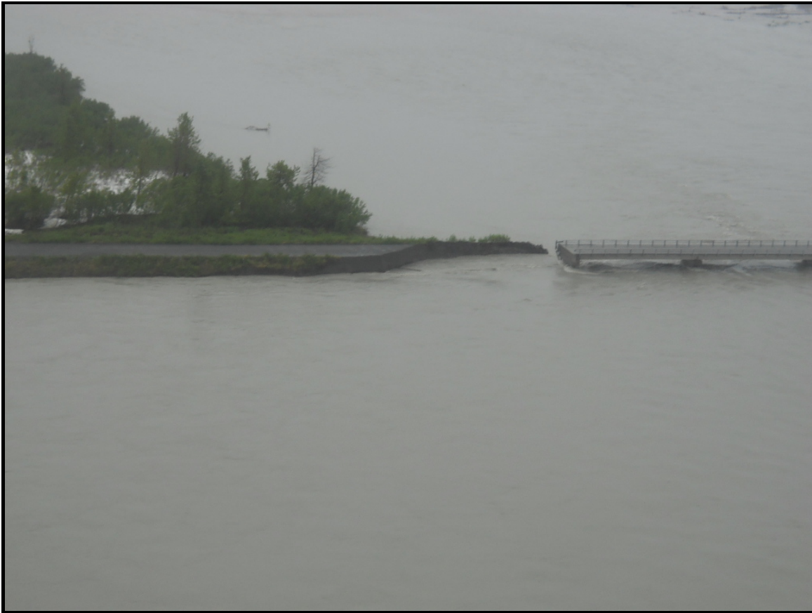
Figure 3 – Bridge 339 looking south at the east abutment June 26, 2012
