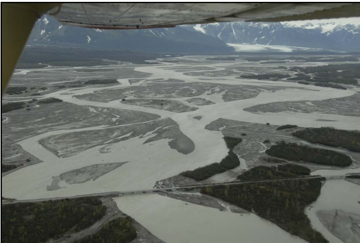
Figure 4 – Bridge 339 looking north September 29, 2008
