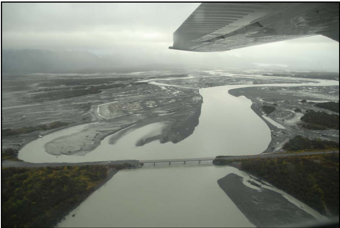
Figure 2 - Bridge 339 looking north October 6, 2011
