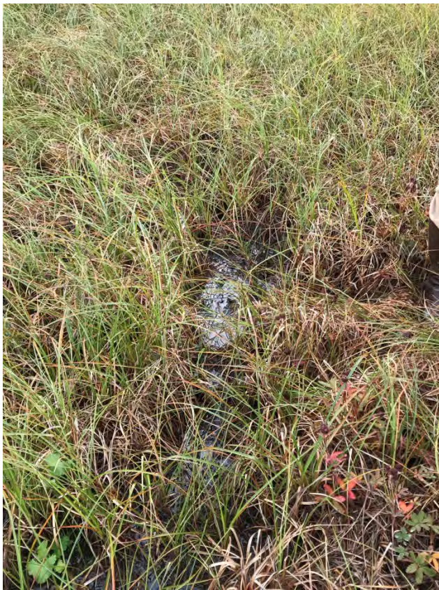
Photo 4: Indistinct channel/seepage flow at crossing site 1.
